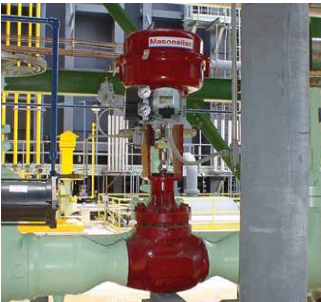
SVI II AP on severe service valve
