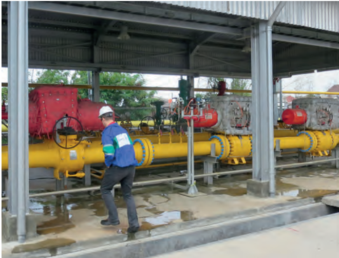
Construction of gas pipeline for Kalimantan Jawa Gas, Indonesia
