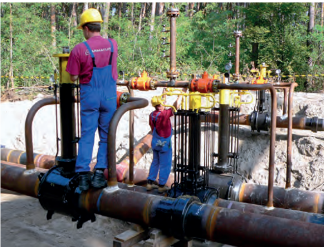
Installation of underground ball valves for Nafta a.s., Slovakia
